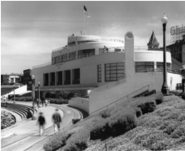
WPA-built Aquatic Park casino, San Francisco. Photograph by Robert Dawson, 2004.
